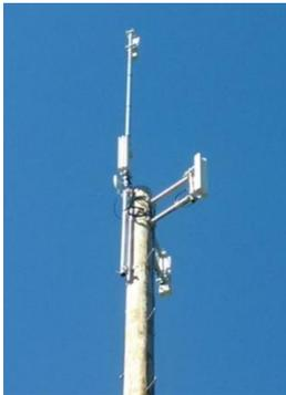
**Figure 1: Antennas on top of 50' pole in Royalston.**
